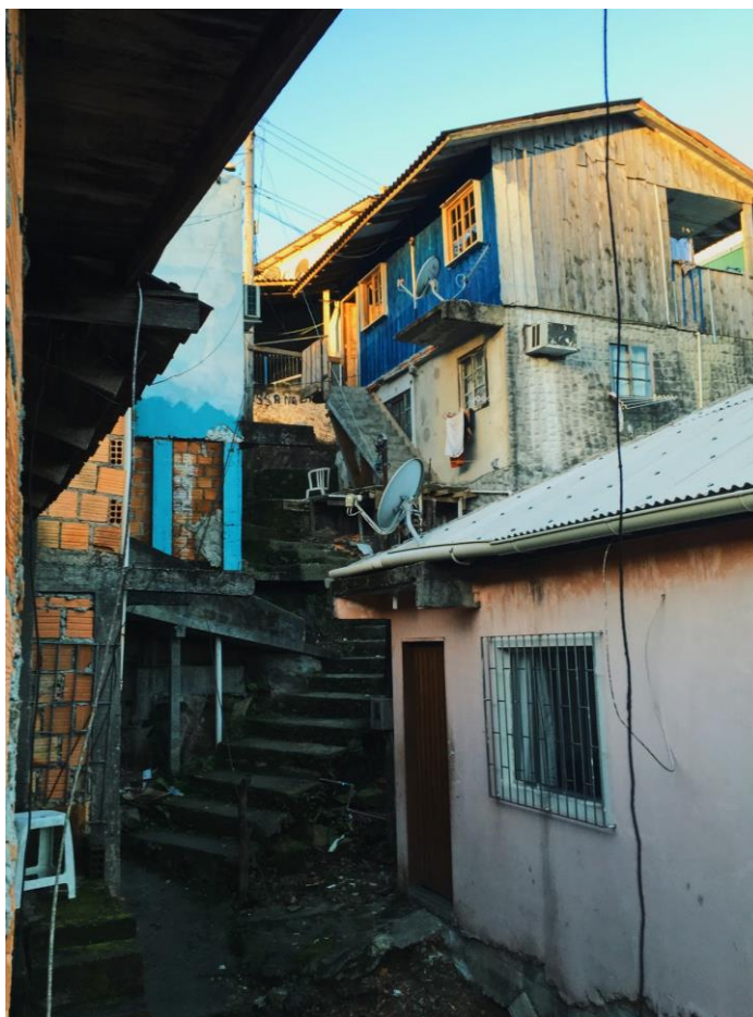
Figure 5: A staircase and houses near Ana and Tiago’s house. Layouts like these both hinder police from entering and allow a drug presence to proliferate.
